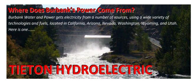
Located on the Tieton River near Yakima in eastern Washington, the Tieton project is rated at 14 megawatts (MW) generated by twin 7 MW hydroelectric turbines.
