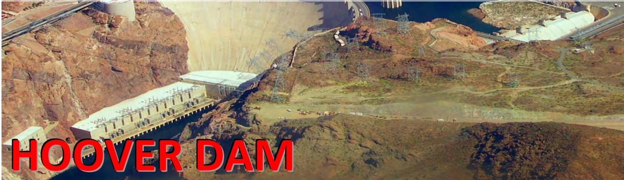
Few power generation facilities are as iconic or inspire as much awe as the Hoover Dam. First envisioned in the early 1900s and constructed between 1930 and 1935 during the Great Depression, the Hoover Dam produces power using 17 hydroelectric turbines rated at 2,080 megawatts (MW) in aggregate. Hoover Dam straddles the Arizona-Nevada border, with one set of turbines on the Arizona side and the other set on the Nevada side.
