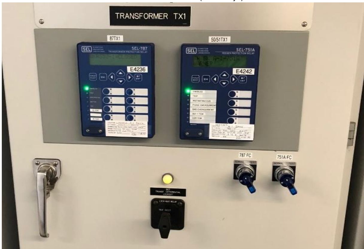
After Installation (New Relays)
