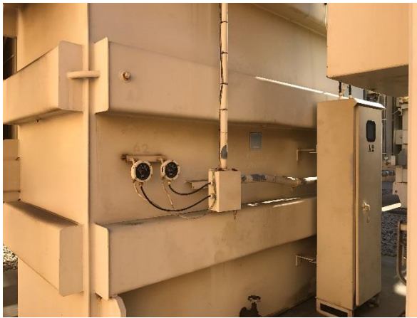
Transformer Bank A-2 Before Installation
