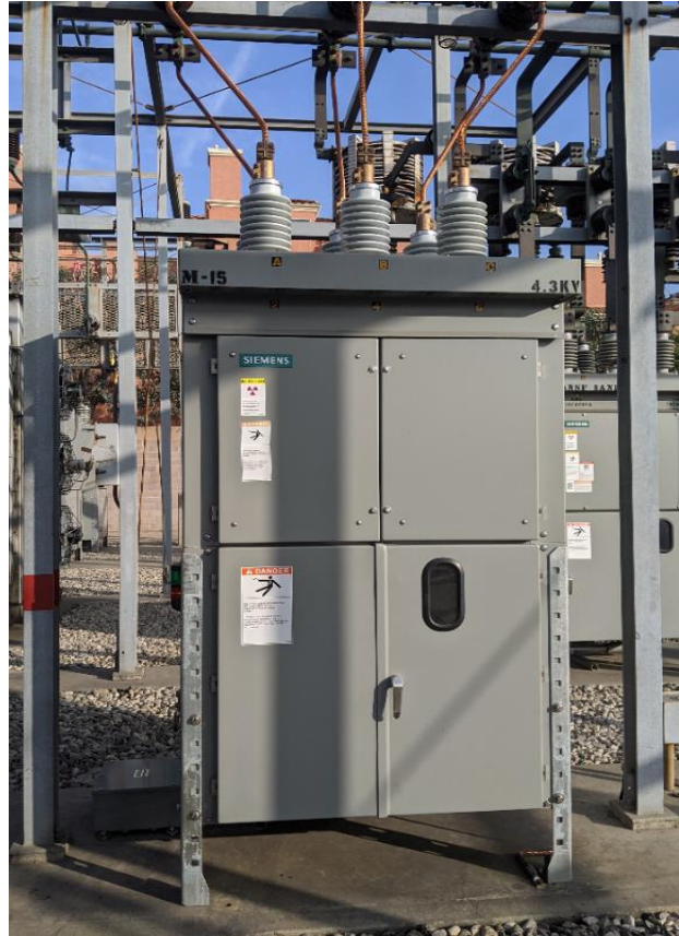
New 4 kV Vacuum Circuit Breaker for McCambridge M-15
