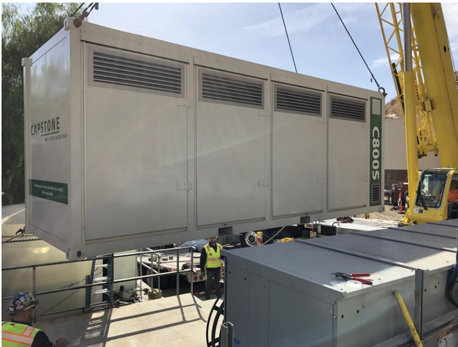
Capstone Microturbine System
