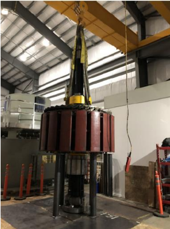
Unit 2 Generator Rotor Inspection
