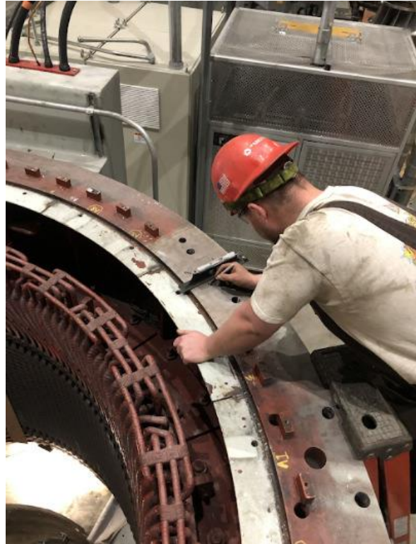
Unit 2 Generator Stator Inspection
