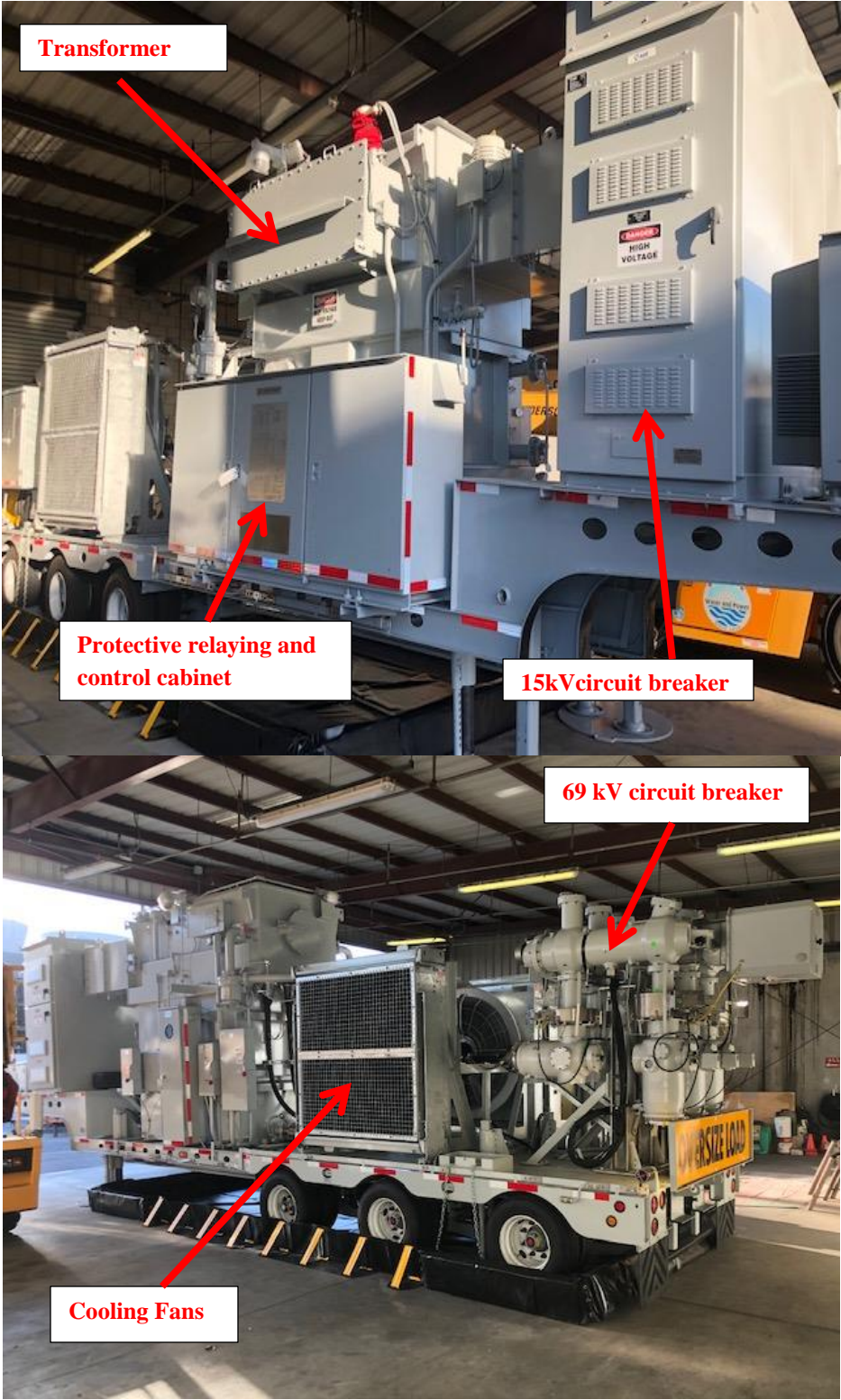
Mobile Substation at BWP Campus
