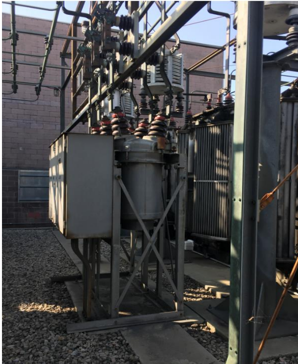
Original 4 kV Oil Circuit Breaker for Flower A-1
