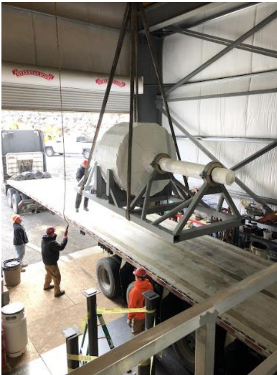
Unit 2 Generator Rotor Transport
