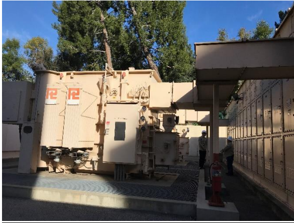
Transformer Bank A-2 Before Installation
