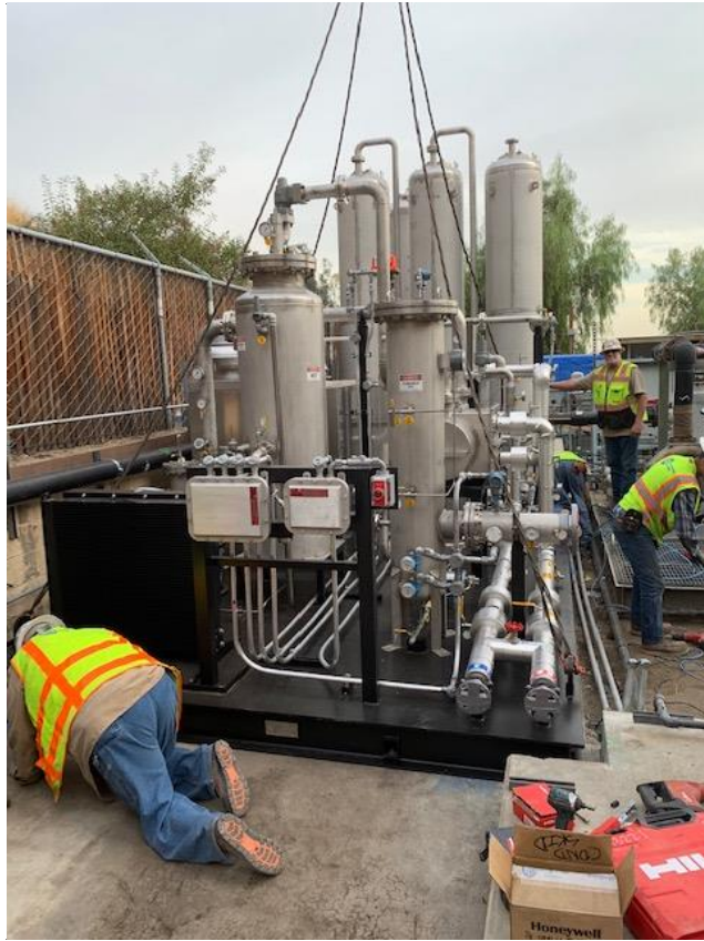
LFG Conditioning Skid
