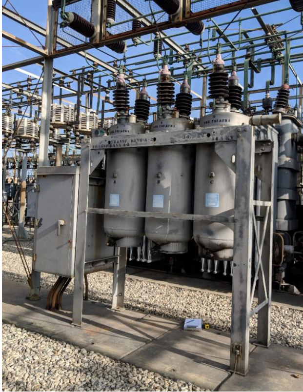
Original 34.5 kV Oil Circuit Breaker for Winona A-2
