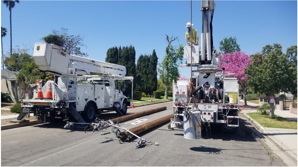
Pole top transformer and arm assembly installation prior to crane set
