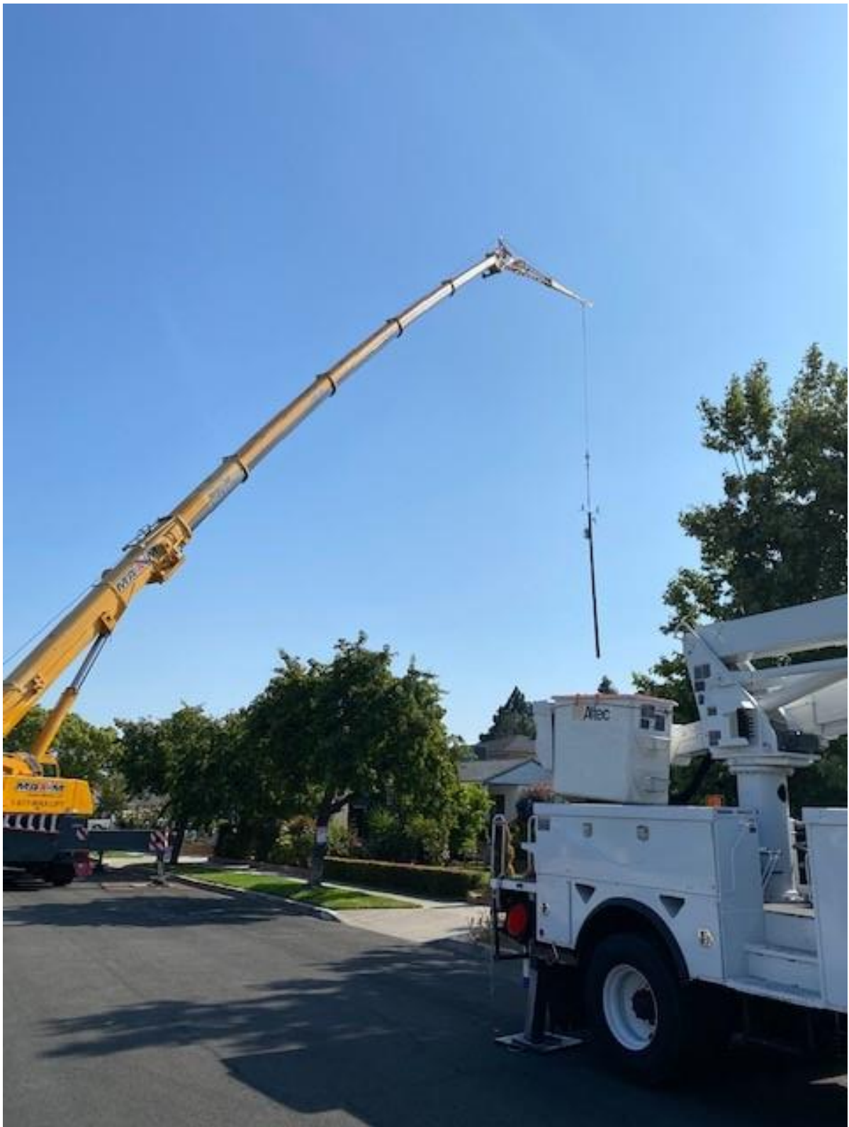
Crane pole setting with transformer and hardware assemblies installed
