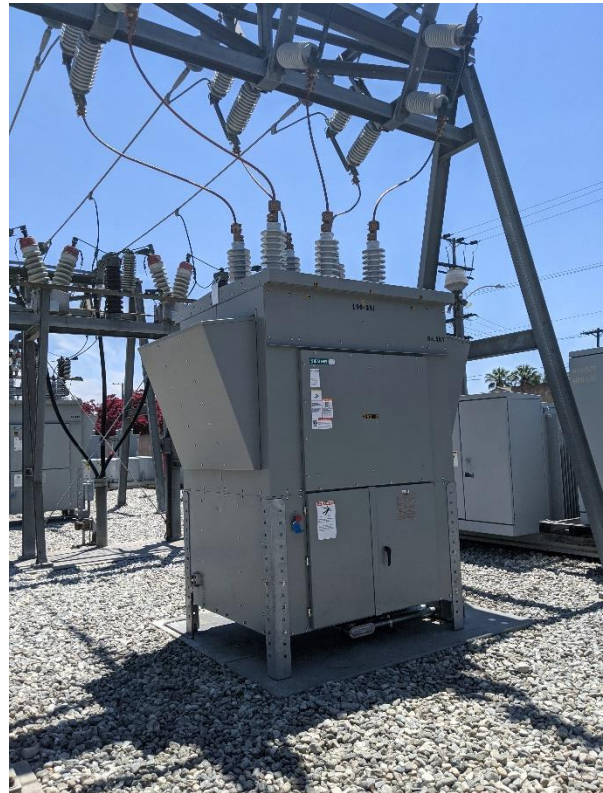
New 34.5 kV Vacuum Circuit Breaker at Lincoln
