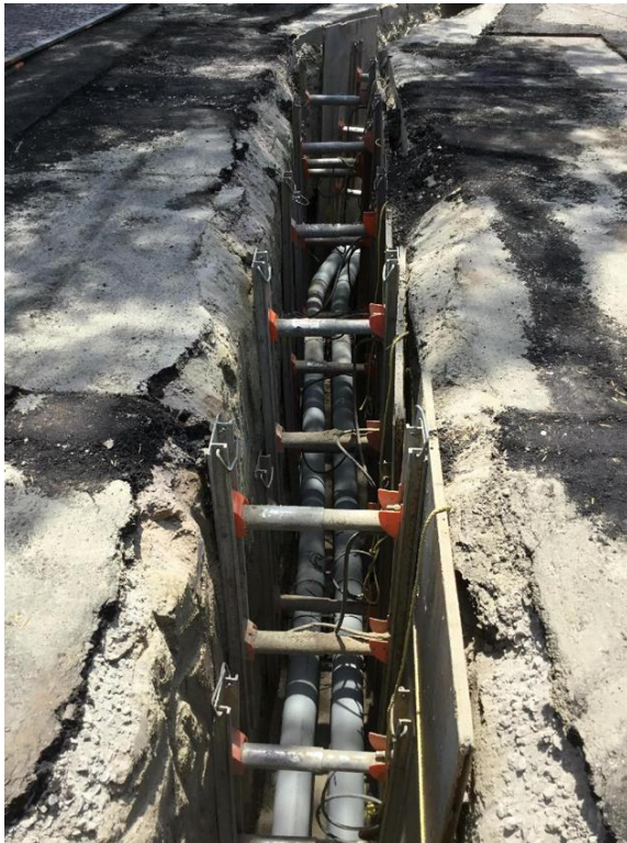
Conduit installation on California St.
