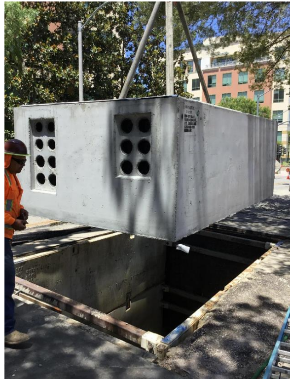
Manhole installation on California St.
