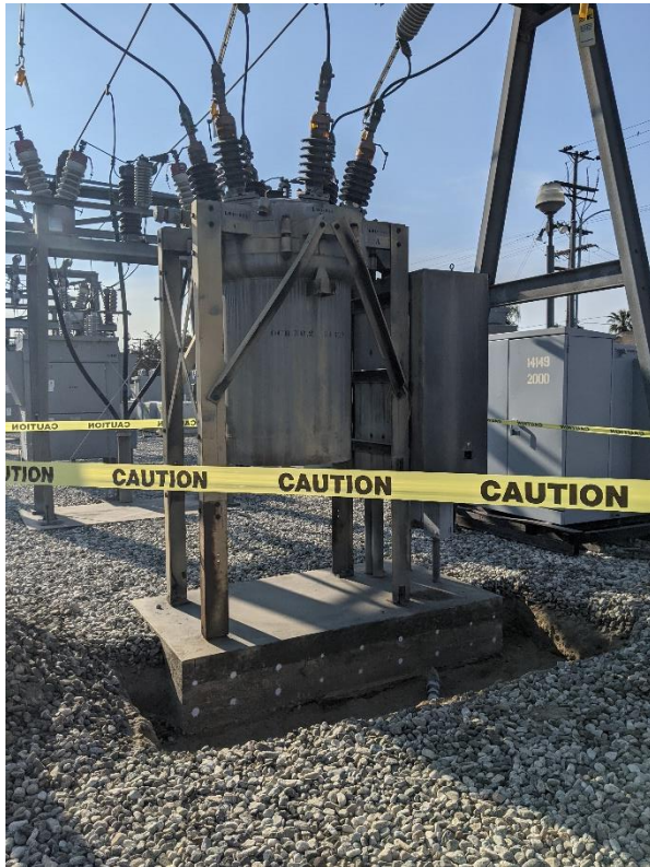
Original 34.5 kV Oil Circuit Breaker at Lincoln
