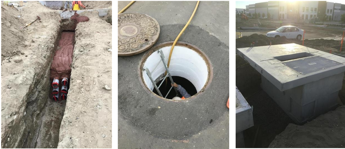
Figure 2 - Underground electrical substructure installations on the project site
