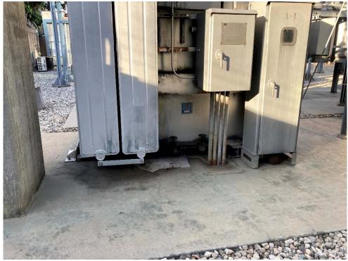
Photo 13: A small transformer oil leak was present below the southernmost transformer. The leak was old, controlled with absorbent, and did not extend beyond the concrete pad.
