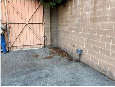
Photo 11: A stormwater drain was blocked with leaves in the northeastern corner, inside the vehicle access gate.
