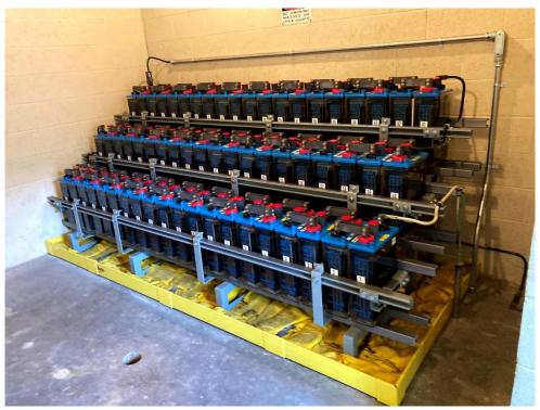
Photo 6: The bank of lead-acid batteries at the southern end of the control house was in secondary containment. A small bathroom was located between the control room and the battery room.
